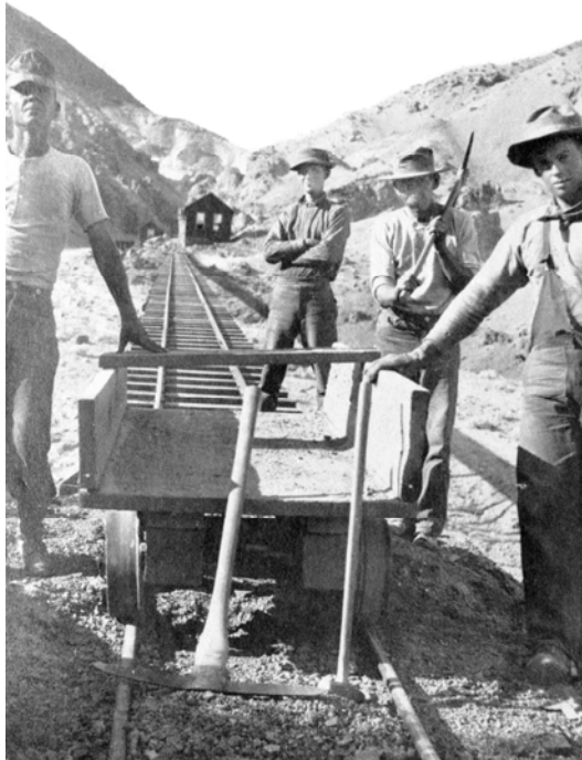
Working on the Borax Properties Limited mine railroad,
