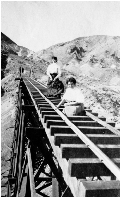
These two dare devils pose on the newly completed trestle.
