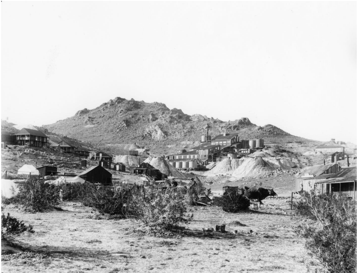
The Exposed Treasure Mine early 1900s, Standard Hill, Mojave Mining District. Photo by C. C.
