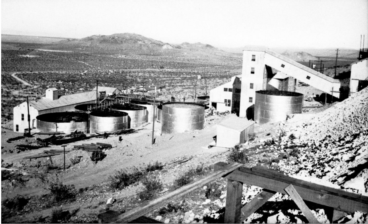
California Geological Survey Photo. "Golden Queen Mining Co. New 300-ton mill and cyanide plant. Photo by W. W. Bradley." Tucker, 1935, p. 477.
